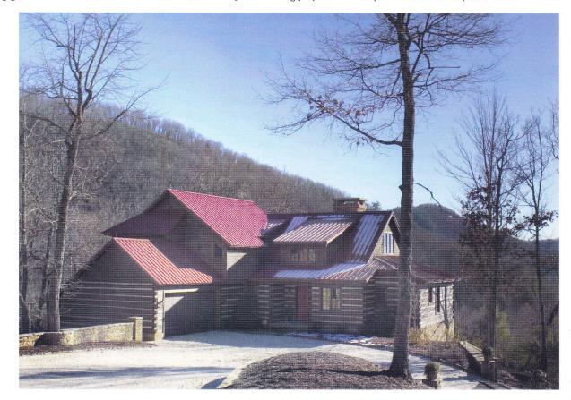
RIGHT Special care was taken to harvest no live trees for the home's exterior; its split log construction provides "thermal lag" which, enhanced by the air-tight sandwiched insulation, enables the house to hold its temperature very steadily in all kinds of weather.
